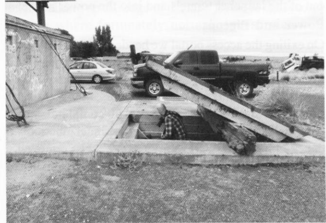
The original personnel entrance to the site, with dubious wooden support
